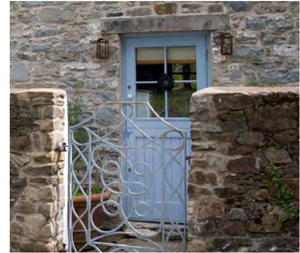
Above: attractive timber door of a traditional, simple style enhances this Gower cottage
