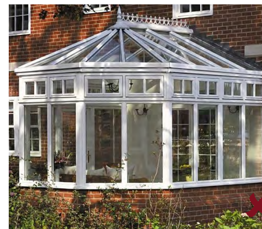
Below: Inappropriate style and choice of material for a conservatory within Gower
