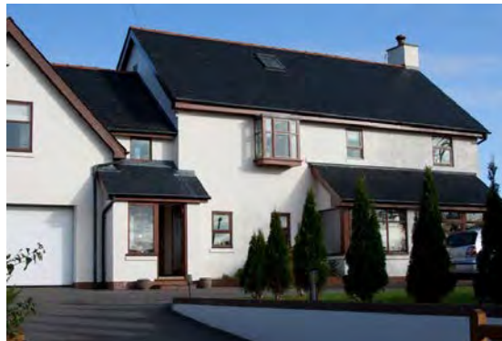
Above: after renovation
