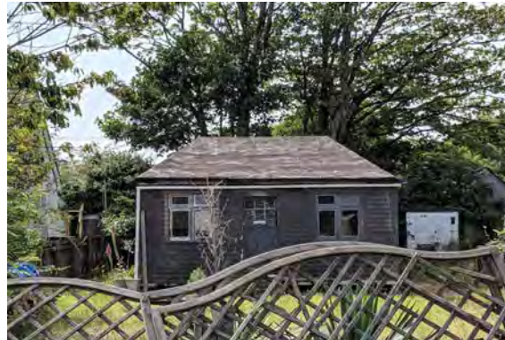
Below: Chalet at Sandy Lane
