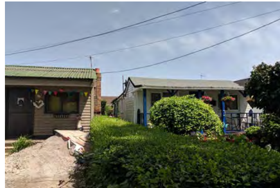
Below: Chalet at Miles Lane
