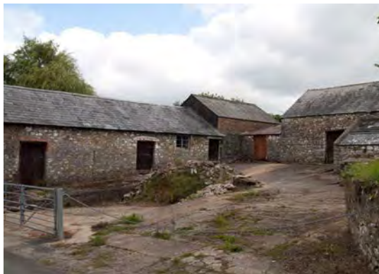
Below: farm buildings used as basis for the preparation of illustrative examples (right)
