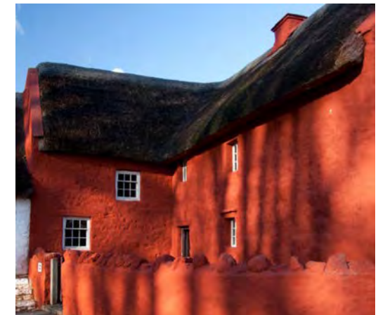
Below: Kennexstone Farmhouse was originally covered with a limewash coloured with ox-blood
