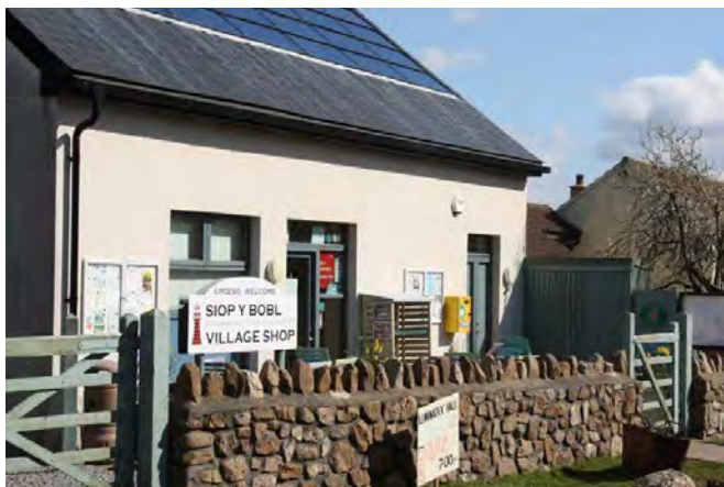
Above: Llanmadoc Village Shop
