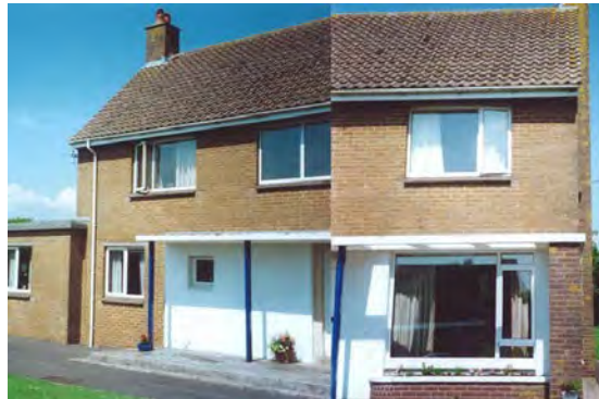
Above: before renovation
