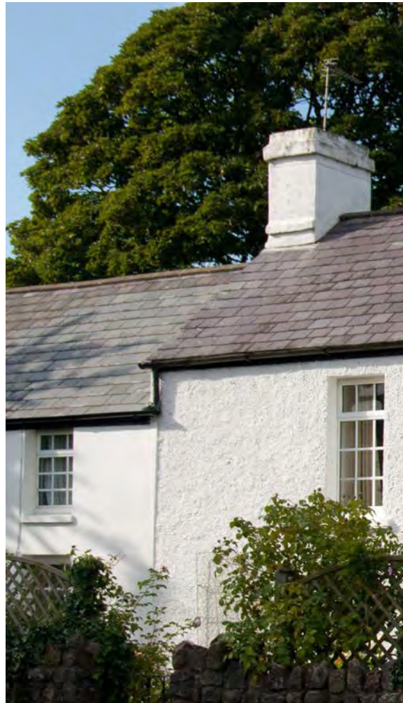
Above: Characteristic smooth and roughcast render finishes, Oldwalls
